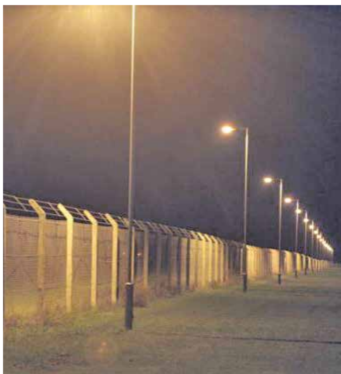
Perimeter lighting on 8m columns
