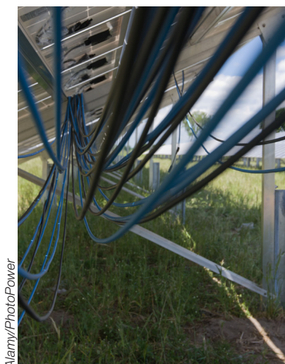
Figure 2: The inverter cables cut at each end by thieves for removal
