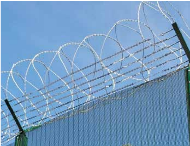
Fig 3. Welded mesh fence with barbed tape topping
