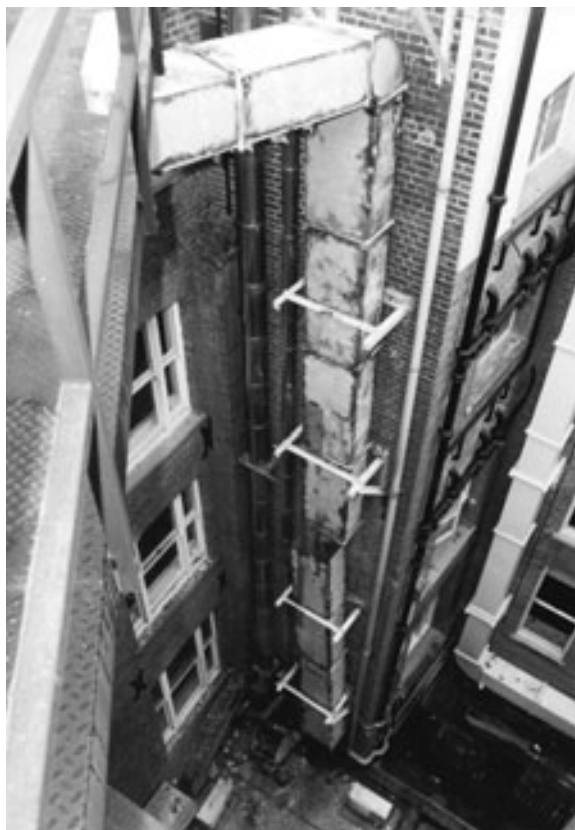
Figure 7: Broken ductwork
