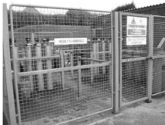
Gas cylinder compounds should be secure and prominently signed
