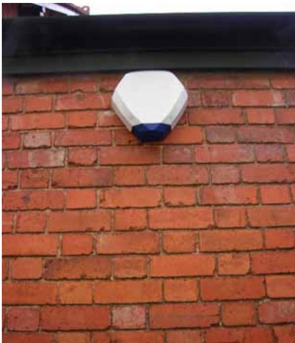
**Fig 4: The external WD should be sited out of easy reach**
